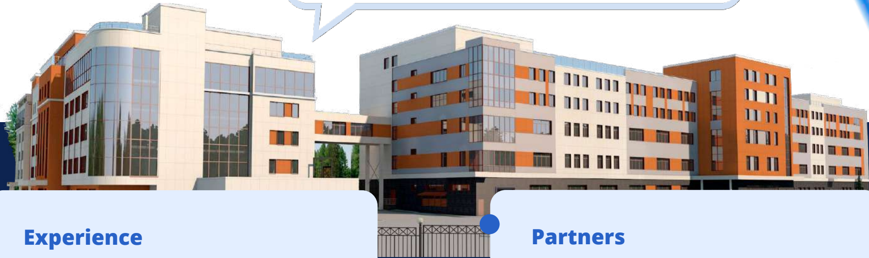
Manufacturing complex in Novosibirsk
